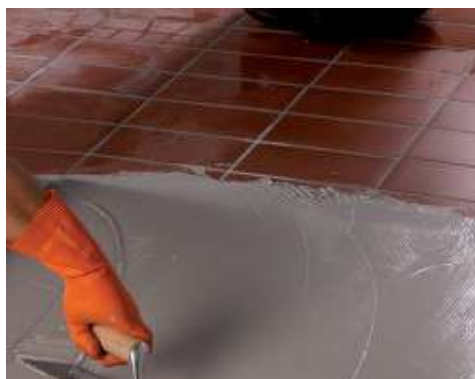
Applying a second layer of Monolastic on Mapepet 150
