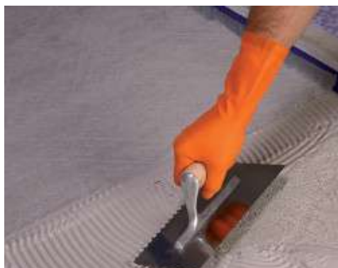
Applying a first layer of Monolastic welded with Mapetex Sel on a new screed
