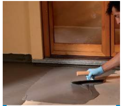
Waterproofing of terraces by trowel
