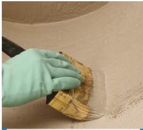
Waterproofing of details by brush
