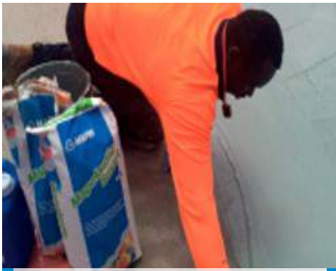
Installing Mapelastic Smart in the 50 metre pool at the Adelaide Aquatic Centre
