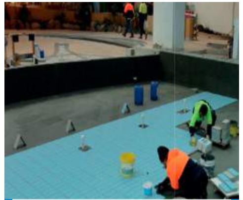
Installing pool tiles over Mapelastic Smart waterproofing membrane
