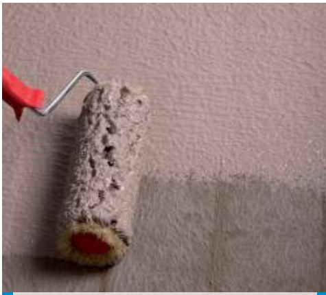
Waterproofing of details by roller
